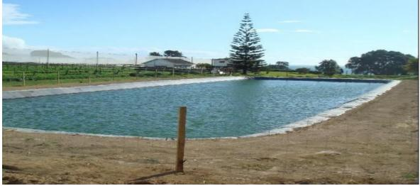
The height from the crest of the dam to the top of the embankment is generally .5 metre which allows for rainfall capture. A building consent is not required for small dams under four metres high with a water volume under 20,000 cubic metres. NZKGI is not aware of a pond exceeding 20,000 cubic metres on a kiwifruit orchard however it is possible. The largest cubic metre area we could find is 11,000.
